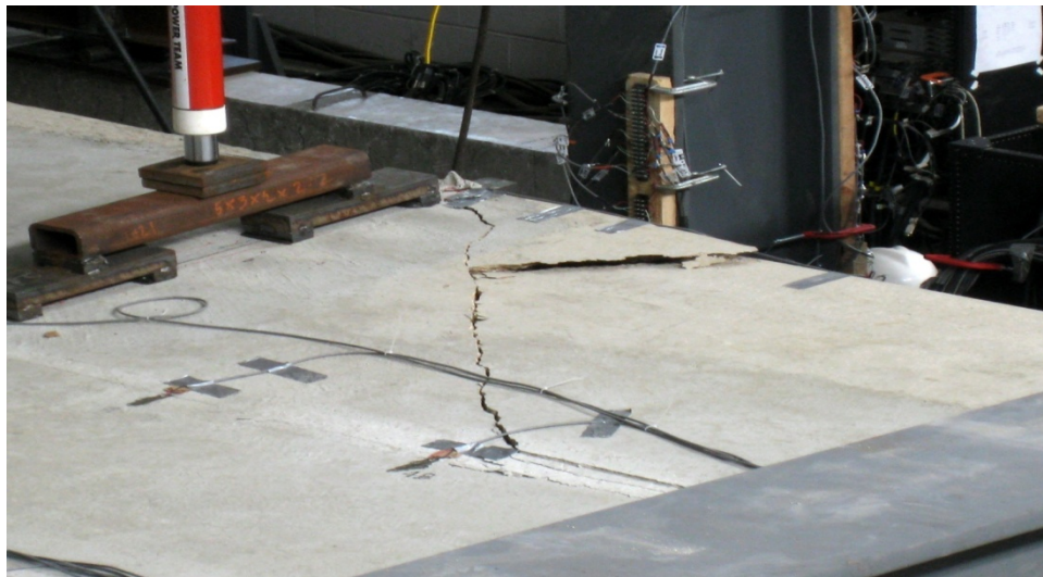
Figure 5: Failure of test specimen was defined by shear cracking of slab
