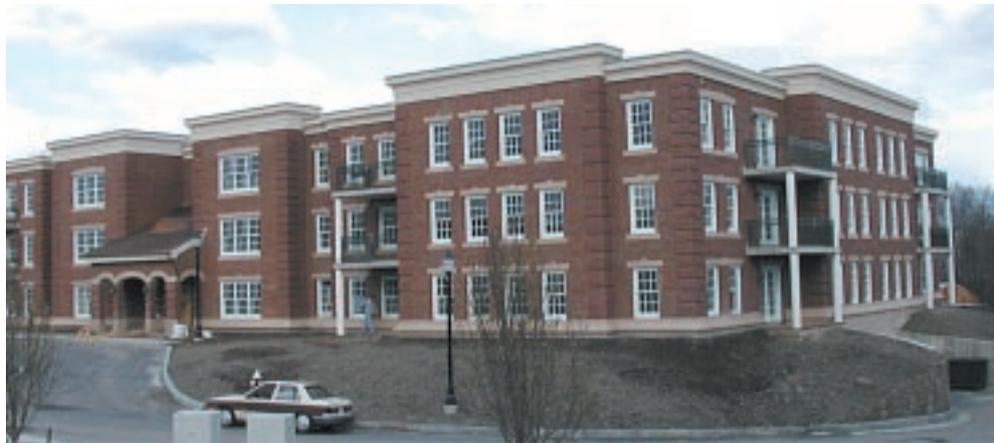
placed the balconies as the steel and precast were being erected. This eliminated the need for a separate crane mobilization to erect the balconies. The quality of precast concrete provides for a long-term maintenance-free balcony.
