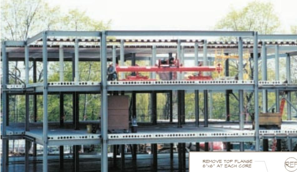
Singly-symmetric steel girders and precast concrete plank proved to be a cost-effective structural system for this Chestnut Hill, MA, condominium.
