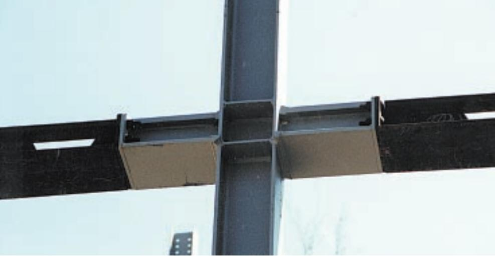
Interior column with "gooseneck" connection welded to both sides of column.
