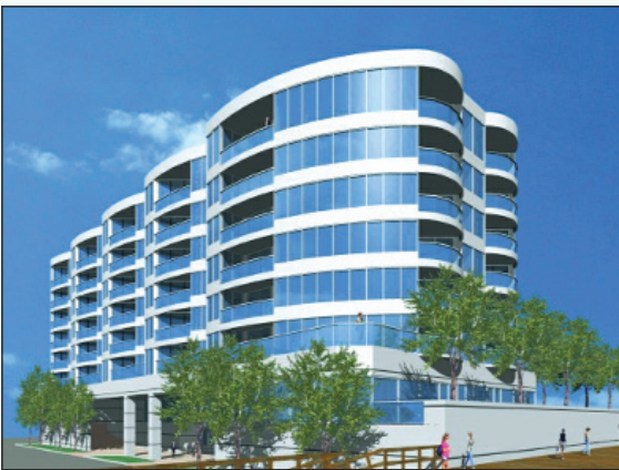
Showing off its curves, the Aqua condominium project under construction in Long Island Beach, N.Y., is employing the Girder-Slab framing system. Rendering: Robert M. Swedroe Architects & Planners; Photo: Canatal Industries Inc.
