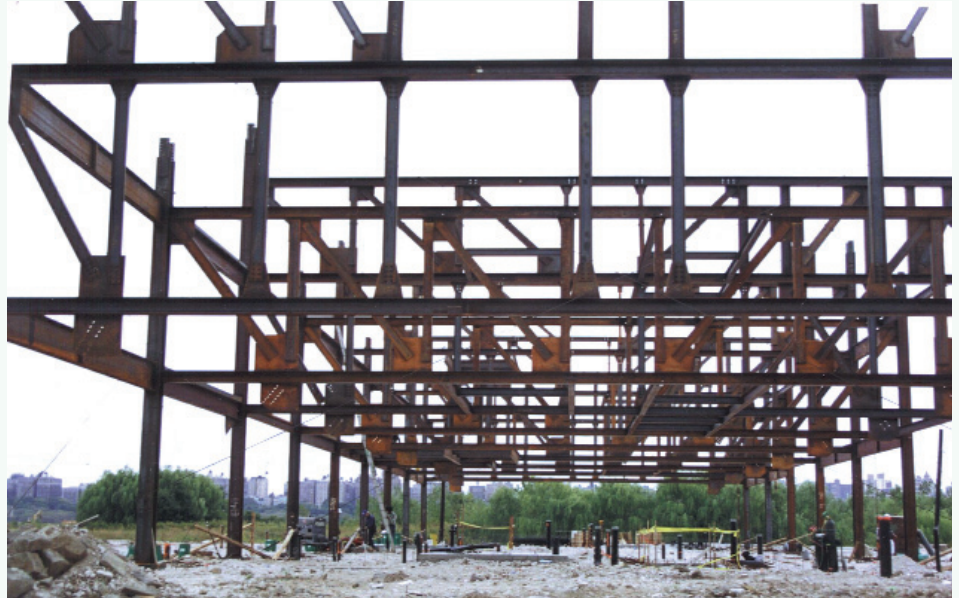
A common ground level view of column-free first floor of staggered truss project.
