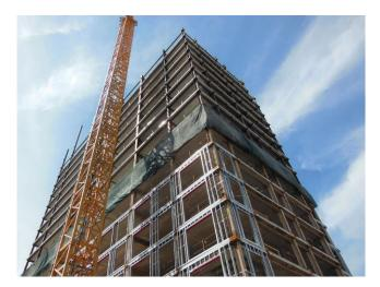
Erection of the 20-story tower, showing the sequence of enclosure on the lower levels during construction of the upper levels.
