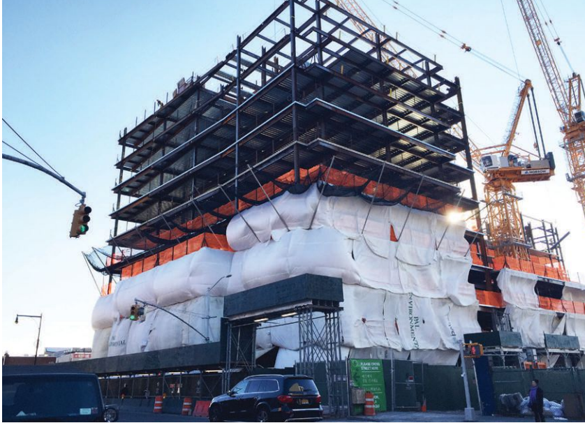
◀ Construction of the 11-story office tower.
