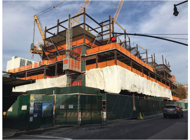
▲ Construction of the residential building.
