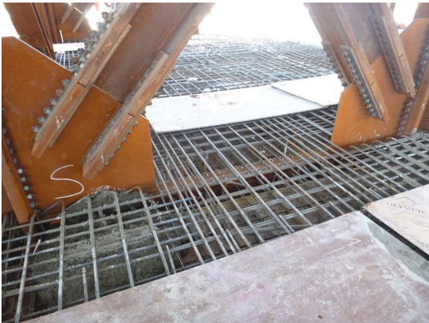
▲ A strap beam erected on-site.
